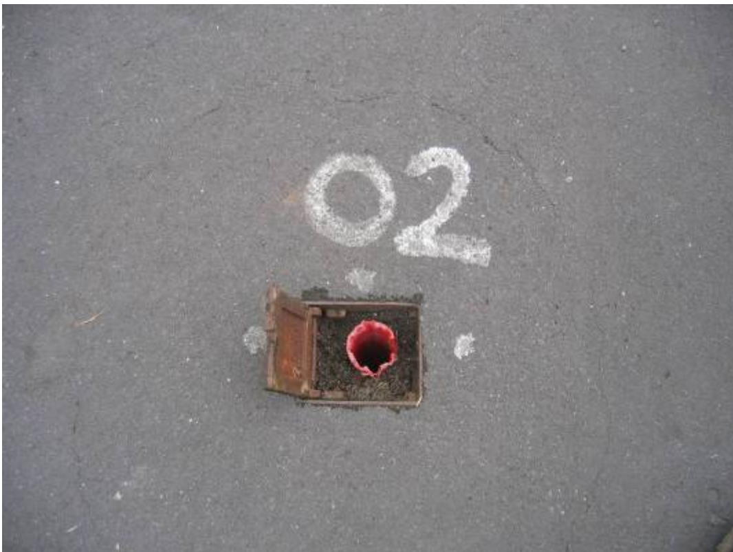
Plate 36 Scarborough South Cliff H4 (AA02)
