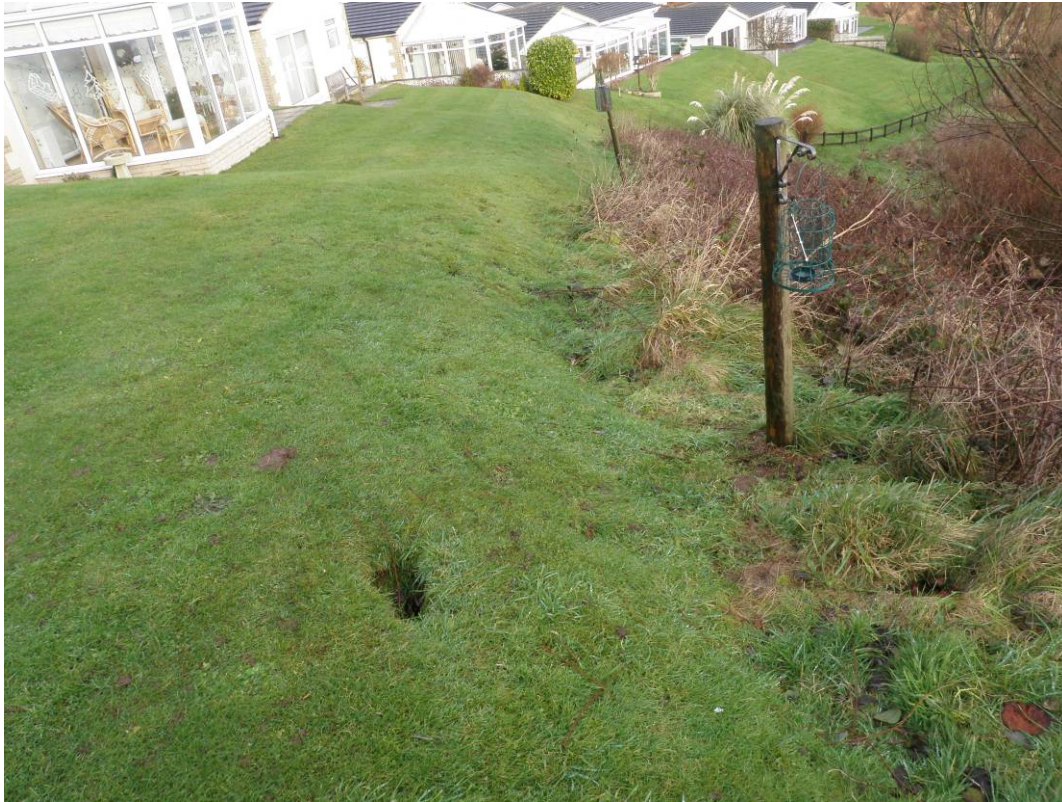
Plate 19 Cliff recession at Knipe Point Headland looking east (13 th December 2010) (Note tension crack development in foreground)
