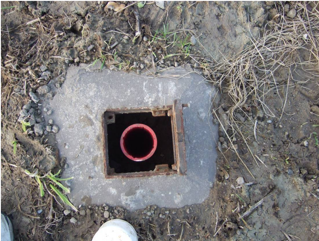
Plate 20 BH21 located mid-slope at Wheatcroft Cliff
