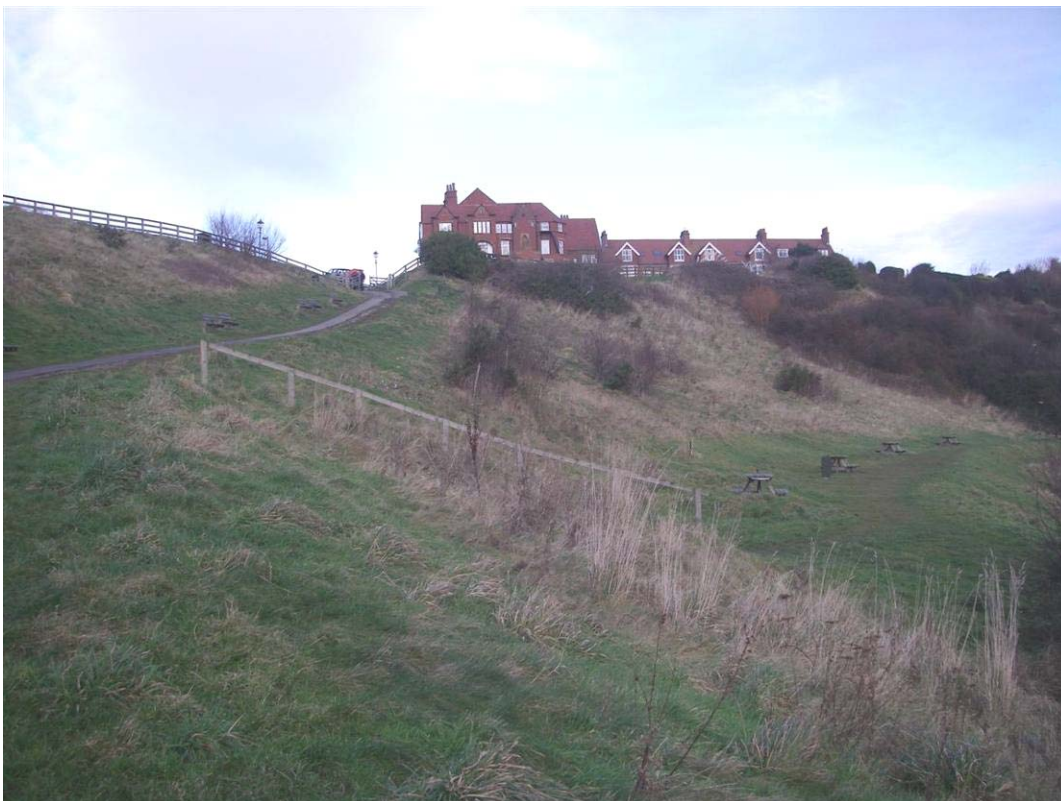
Plate 2 View looking north towards Victoria Hotel from remediated coastal slopes
