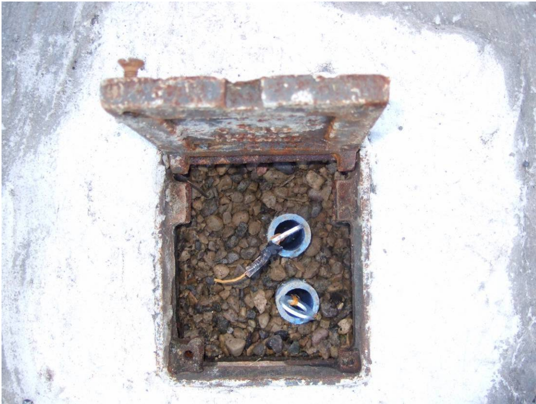
Plate 18 BH19 located on The Promenade above The Italian Garden
