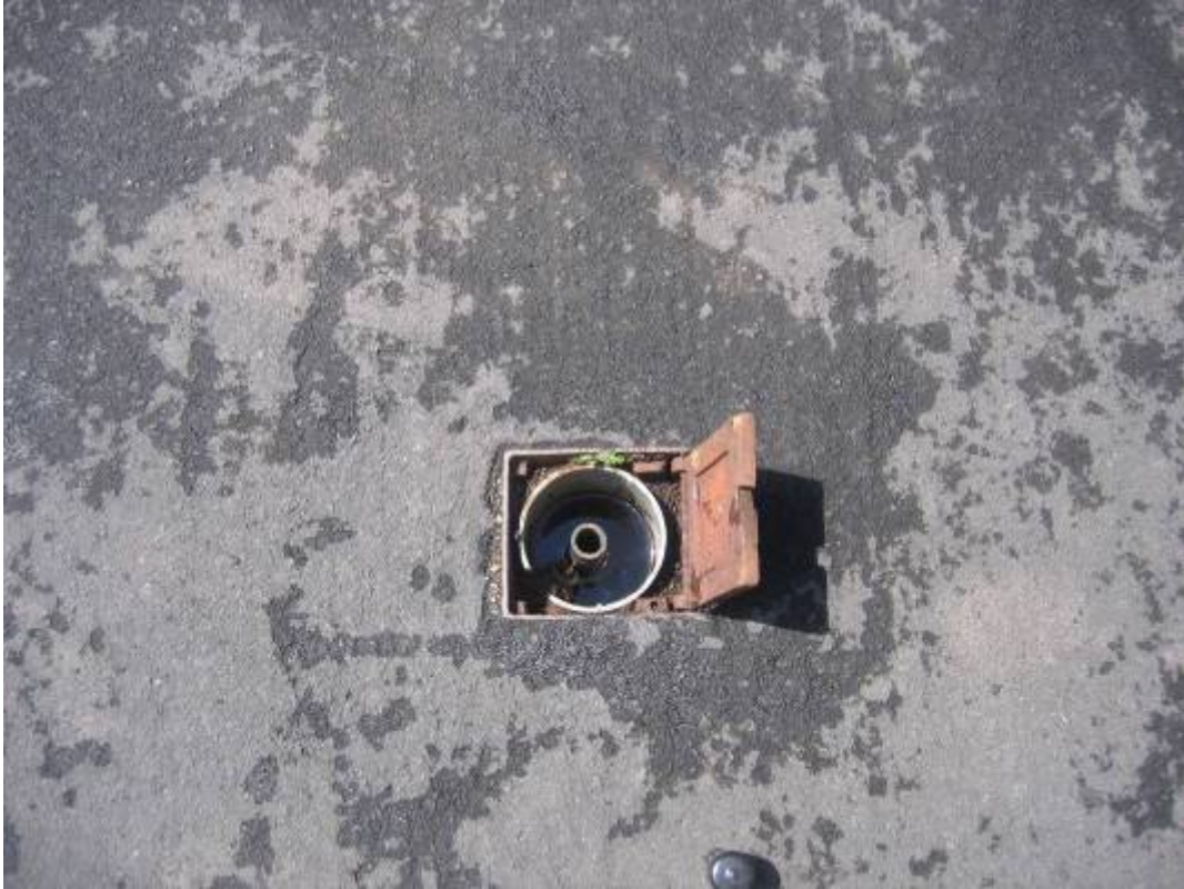
Plate 47 Scarborough South Cliff I2
