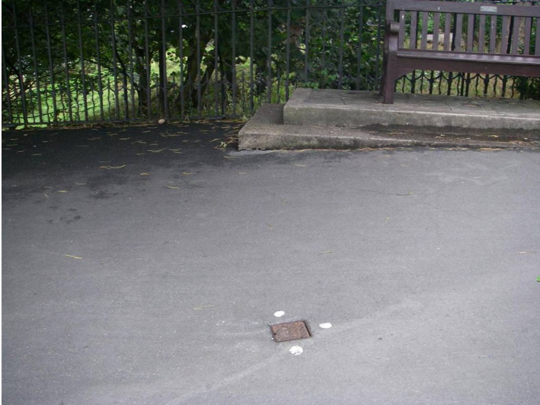
Plate 71 Scarborough South Cliff E3 (AA09) Survey Points
