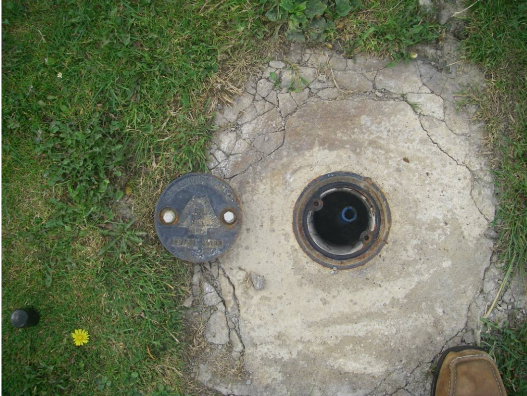
Plate 37 Scarborough South Cliff BH1 SPA (Top)
