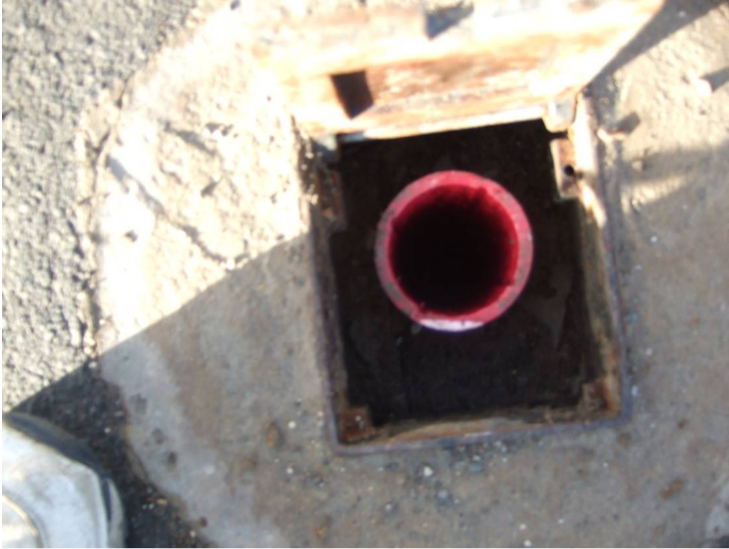
Plate 11 BH12 located on The Promenade above Spa Chalet Cliff
