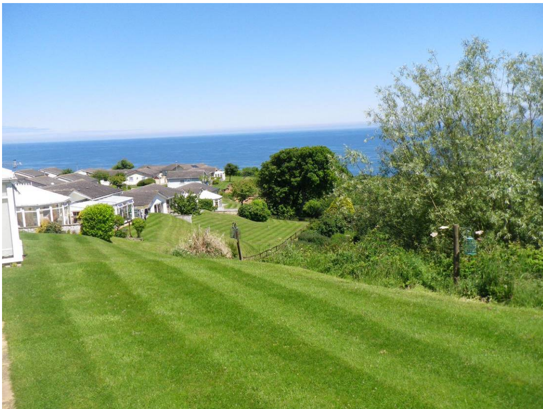
Plate 18 Cliff recession at Knipe Point Headland looking east (17 th June 2010)
