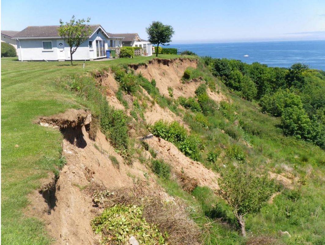
Plate 15 Cliff recession at Knipe Point Headland looking east (17 th June 2010)
