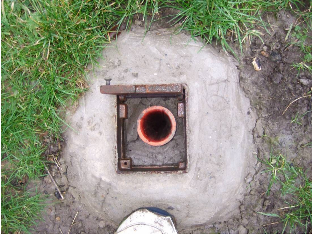
Plate 9 BH10A located at The Holms, Scarborough North Bay
